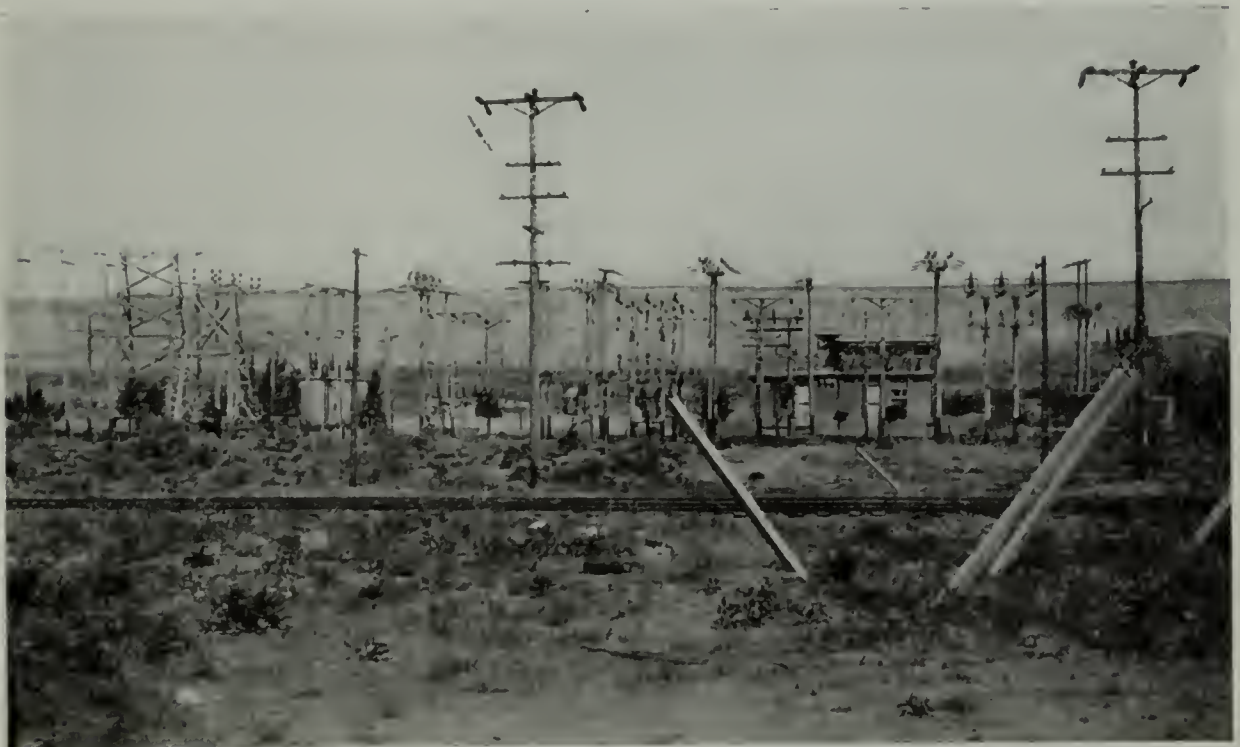
Hanford Substation in the year 1927
